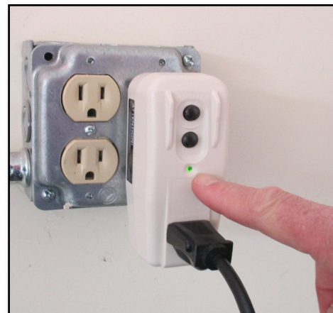
Figure 18. The green light on the GFCI indicates the circuit is protected.
