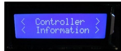
Figure 9.7 Final screens on the K500 Controller
